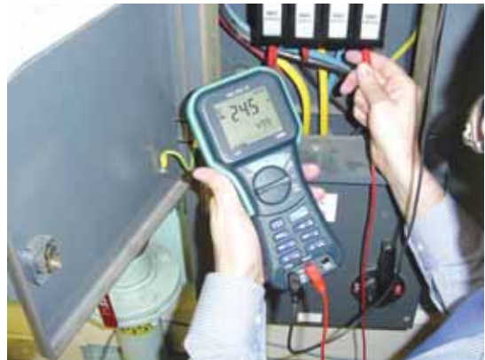
Checking the circuit continuity by multimeter
