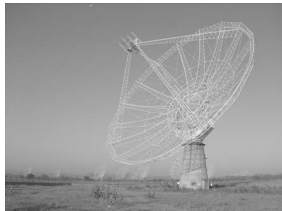
Fig. 3.8 Fully steerable 45 m paraboloidal dishes of the Giant Metrewave Radio Telescope (GMRT) in Pune, India. The GMRT consists of 30 dishes of 45 m diameter with 14 antennas in the Central Array. [Photograph courtesy: Professor Govind Swarup, GMRT, Pune. A color photograph of the above figure appears as Fig. 2 in the prelim pages].
